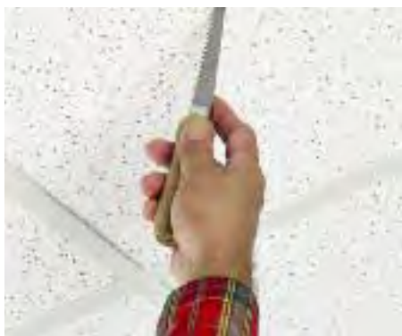
1 Cut 4-1/16" x 4-1/16" hole in ceiling tile.
