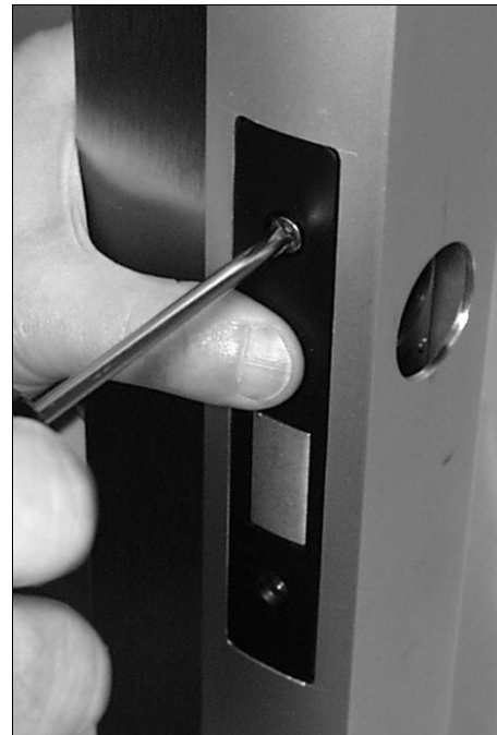
Fig. 4d: Install the deadbolt face plate
