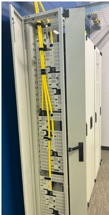
Side view(s) of 150mm VCM with ingress/egress plates installed
