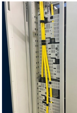
Side view(s) of 150mm VCM with ingress/egress plates installed
