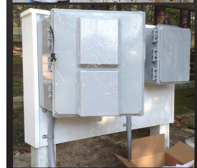
Installer made mounting surface
