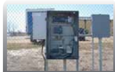
Along a gate using metal tubing to run wiring from one enclosure to another
