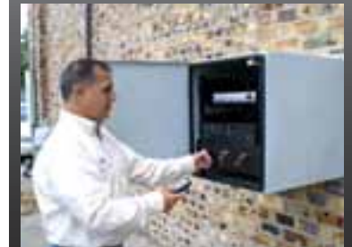
Rack Enclosure mounted on a wall
